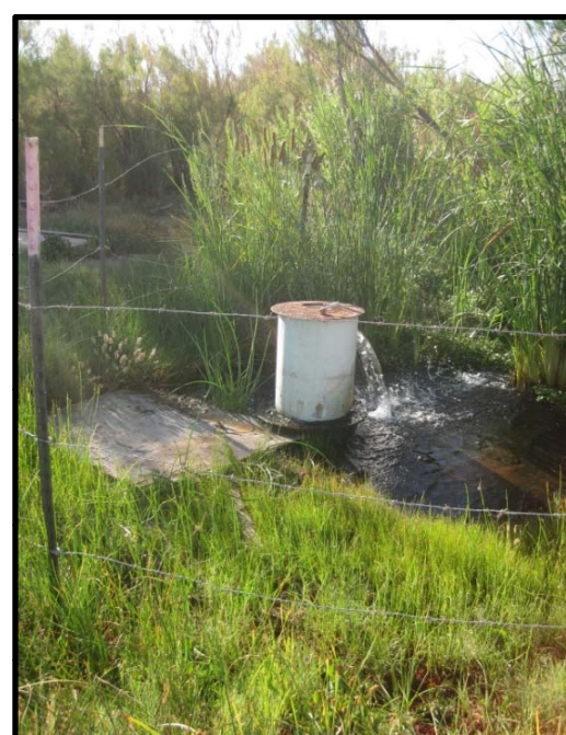
Close-Up Photo of Bartlett Well Showing Flowing Water
