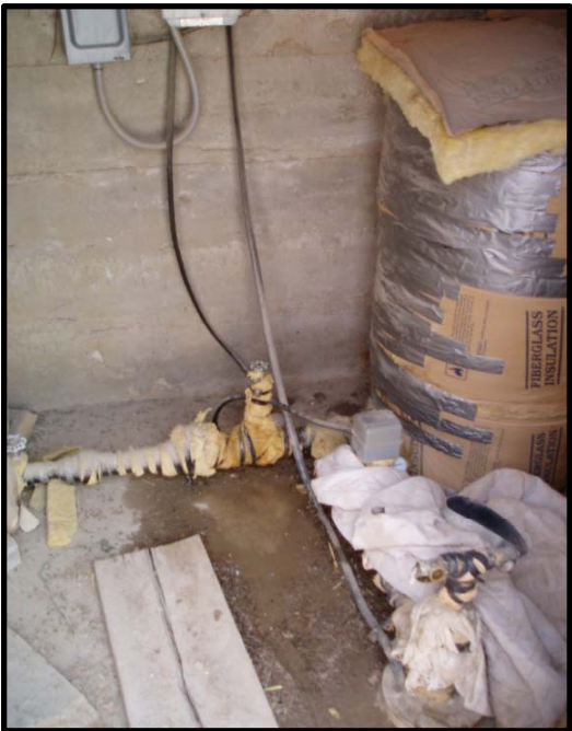
Dolomite Well Inside Well House
