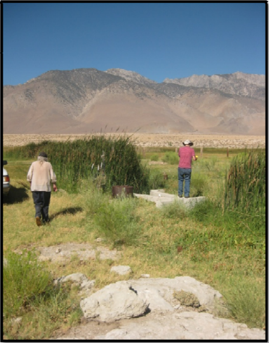
View to the West of Cottonwood Flume (Note that the concrete structure is the flume used to gauge flow)
