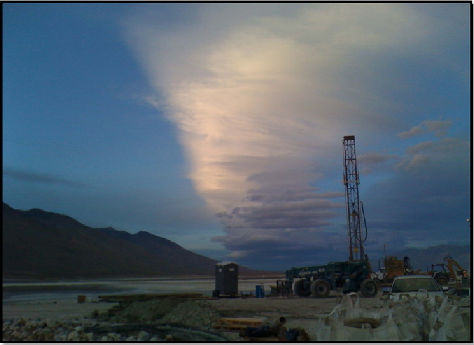
Installation of Monitoring Well at DWP-7
