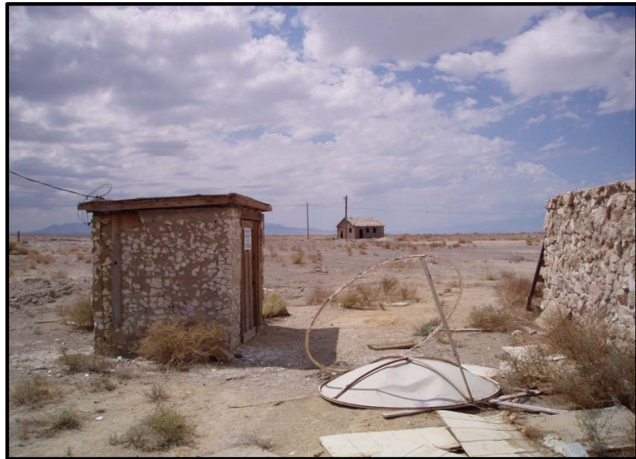
Dolomite Well House
