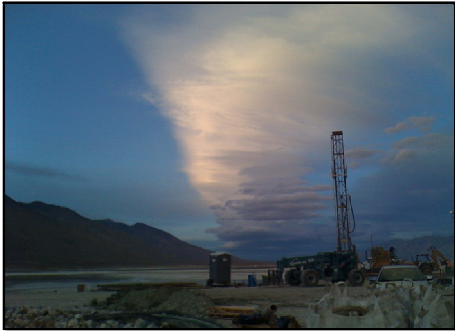
Installation of Monitoring Well at DWP-7
