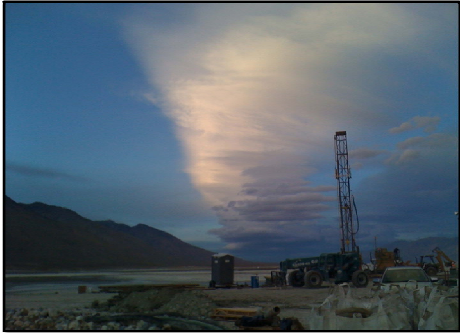
Installation of Monitoring Well at DWP-7
