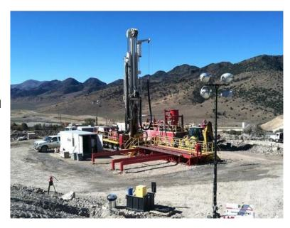
This project requires continuous construction, including night work, to ensure the stability of the boreholes for the groundwater production wells.
