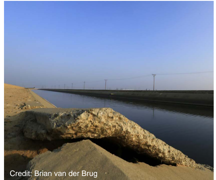
Rupture of Canal in the Central Valley due to Subsidence
