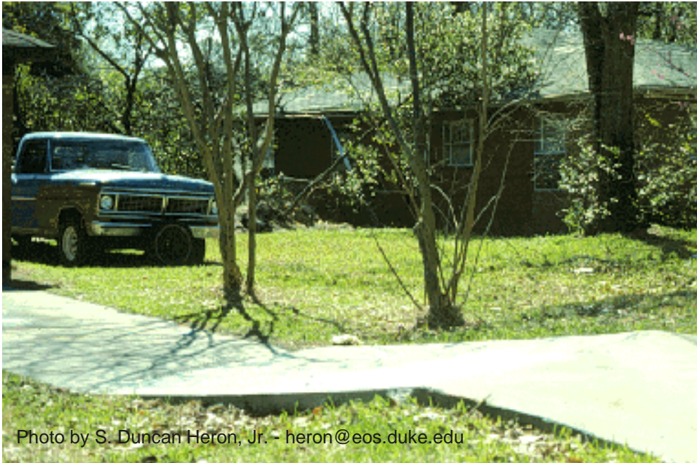
Buckled Sidewalk and Water Well Pump Foundation Pushed Up Relative to the Surrounding Ground By Subsidence
