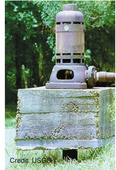
Buckled Sidewalk and Water Well Pump Foundation Pushed Up Relative to the Surrounding Ground By Subsidence
