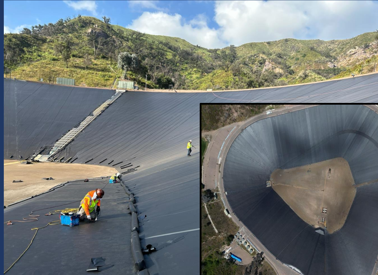
Liner Installation Completed on June 1 , 2026
