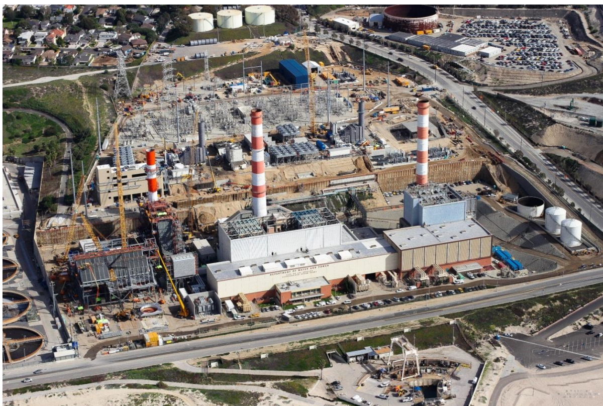
Figure 34: Aerial View of Construction at Scattergood Generating Facility
