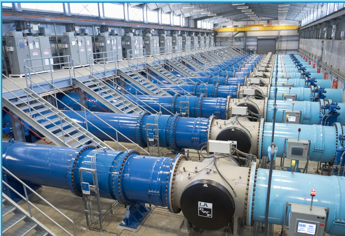
The state-of-the-art Los Angeles Reservoir Ultraviolet Disinfection Plant was commissioned in 2022 and is an important part of LADWP's complex network of water treatment processes at the Los Angeles Aqueduct Filtration Plant. The facility can treat up to 650 million gallons of water per day as they pass through its 15 UV reactors.
