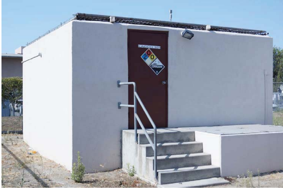
Plate 16: Building 5, Oblique View to Southwest.
