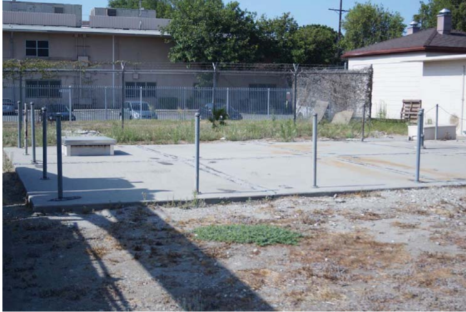
Plate 18: Concrete Forebay and Sand Trap Cover, View South.
