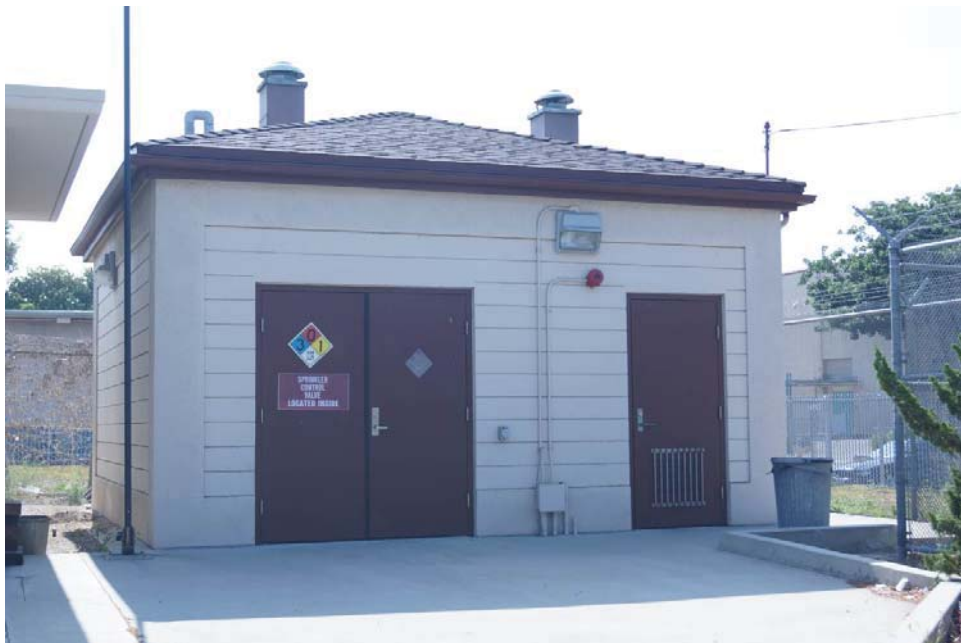
Plate 17: Building 6, North Façade, View to Southwest.
