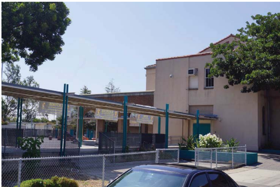
Plate 20: 99th Street Elementary School Building 1, North Side, View Facing Southwest
