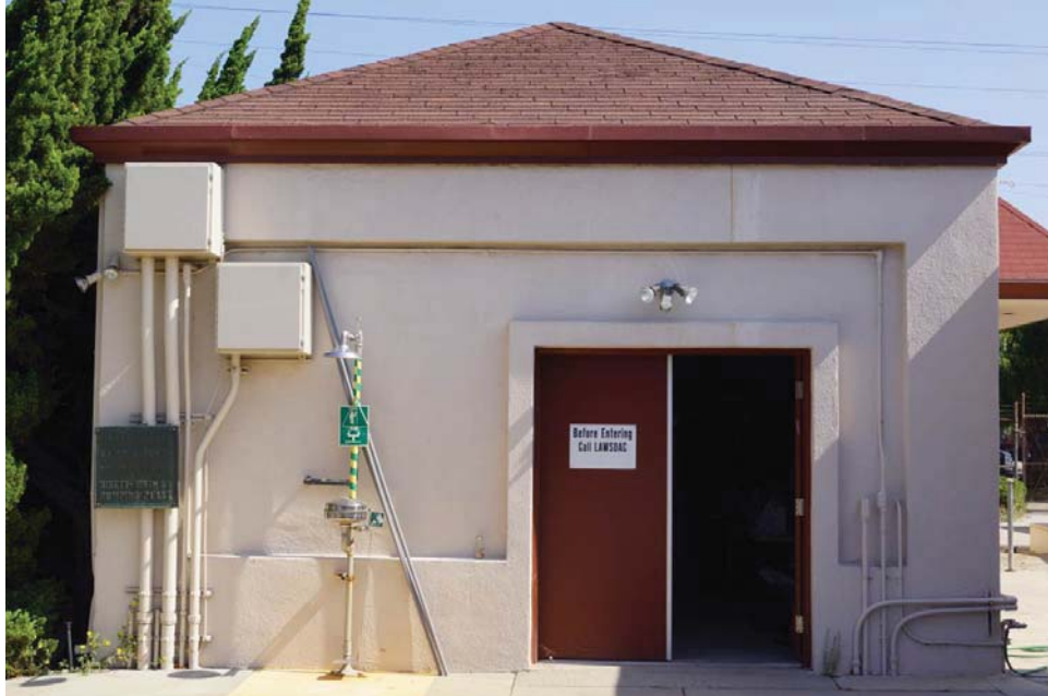
Plate 12: 99th Street Wells Pumping Station Building 1, View Facing North.
