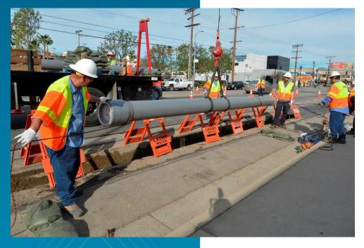
Project Schedule February 2018 -February 2019 Region Encino which will replace approximately one mile of 12inch water mainline installed in 1932 with earthquake resistant ductile iron pipe.
