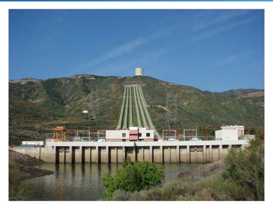
Currently deployed options to deal with overgeneration including storing energy in the Castaic pumped storage plant or selling the energy to its neighbors. Castaic is rated at about 1,175 MW of capacity and is about 70% efficient, meaning it throws away 30% of the energy it stores. Selling energy to neighboring utilities is an important options, but what happens when LA's neighbors are saturated with RE?
