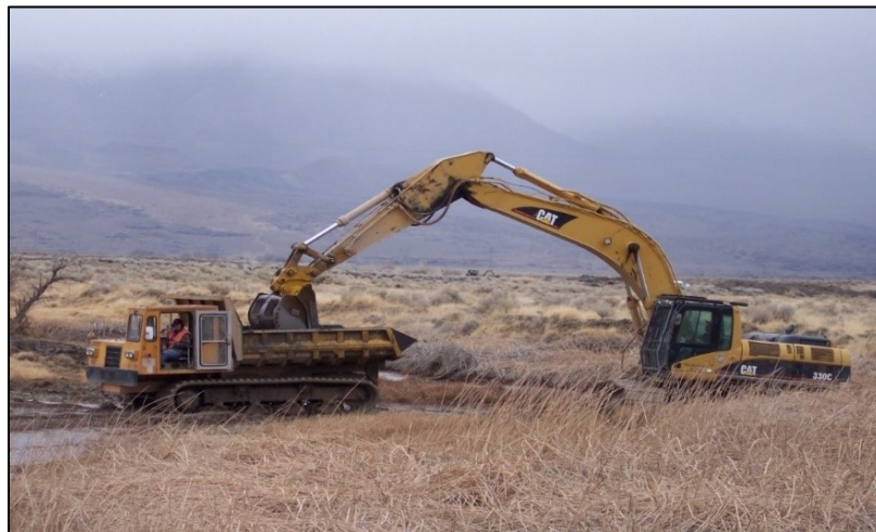
Figure 3. Channel clearing work downstream of the LORP Intake, pre-project
