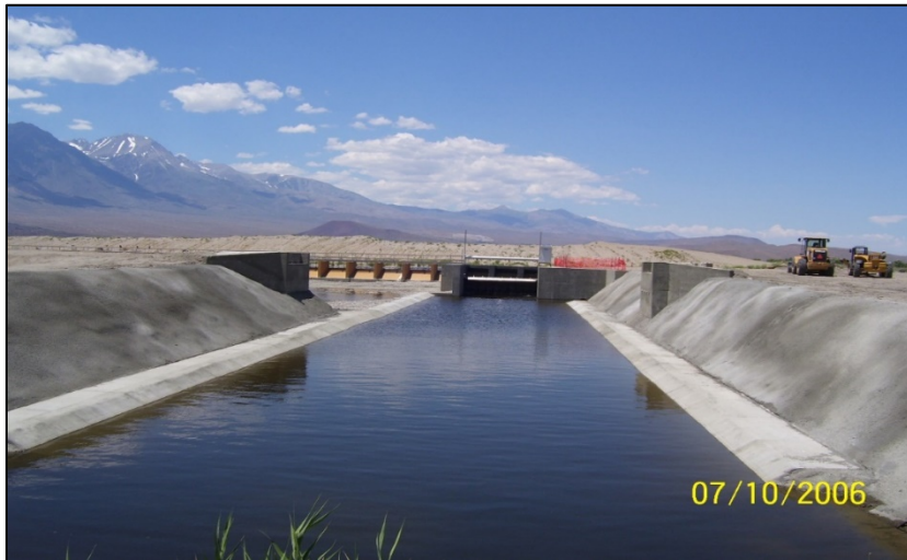
Figure 2. Concrete lined section at LORP Intake, July 2006
