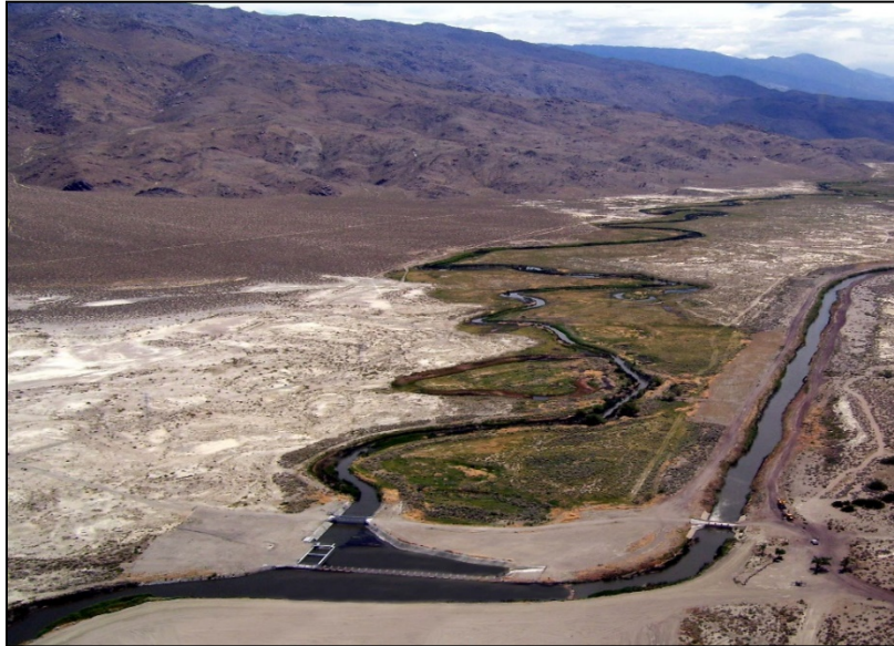
Figure 7. Aerial view of LORP Intake looking south post construction and release of flows
