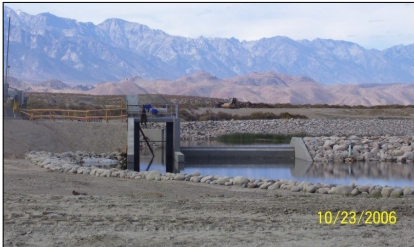
Figure 5. LORP Pump Station Forebay, October 2006
