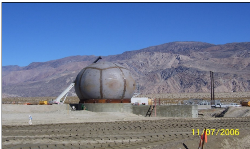
Figure 6. LORP Pump Station during construction, November 2006
