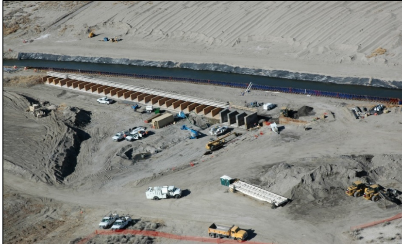
Figure 1. LORP Intake Construction, looking northwest, February 2006
