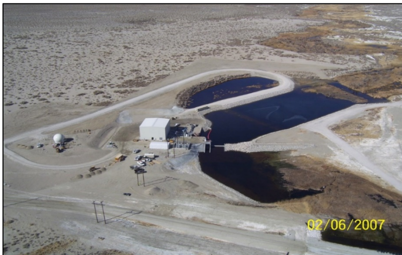
Figure 8. Aerial view of LORP Pump Station looking north following flow release, February 2007
