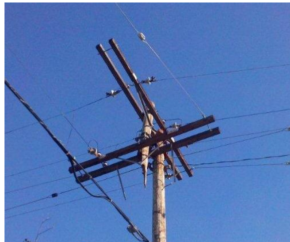
Figure 21: Typical LADWP Broken Wood Pole
