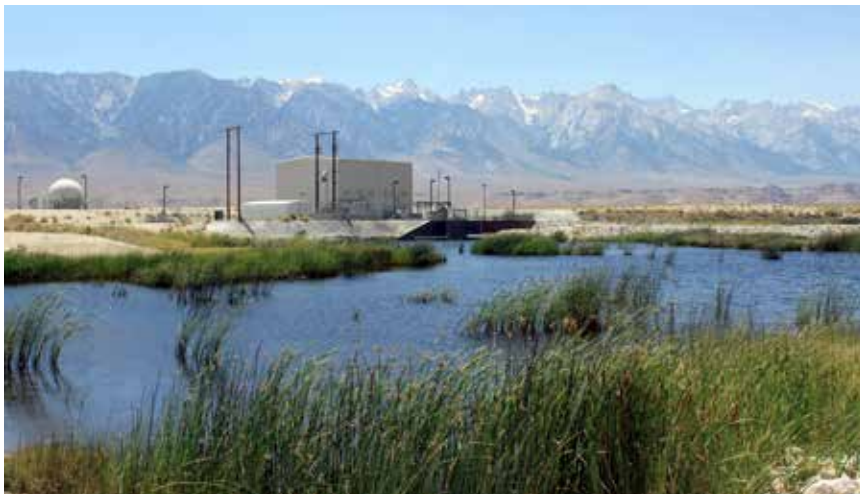
■ LORP Pumpback Station
