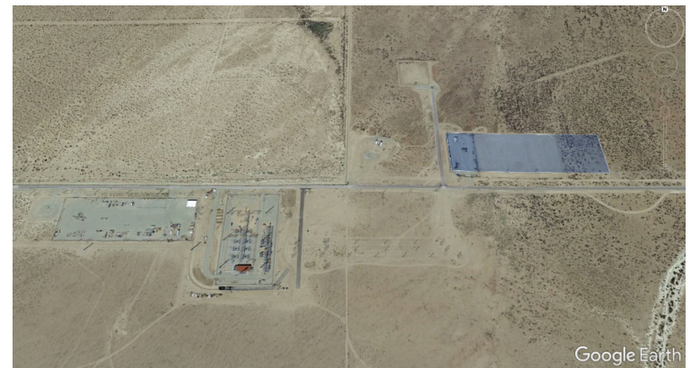
Beacon Site – EPRI Supplemental Bulk Energy Storage Cost and Performance Study
