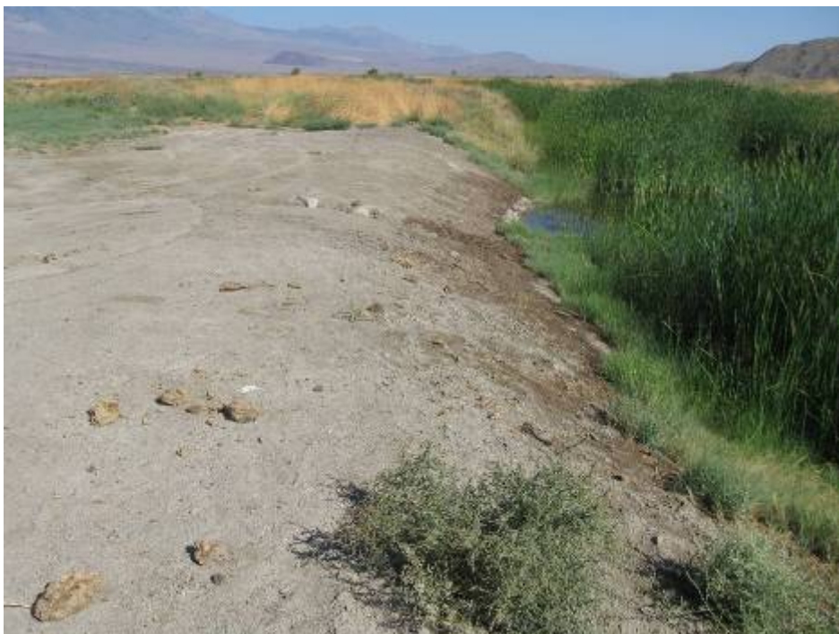
Photo 6. River banks at old road crossing near Blackrock Ditch are still barren.
