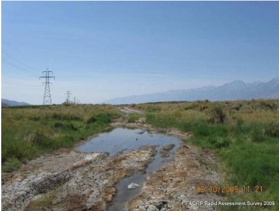
Photo 5. Rehabilitated road near the Intake with some flooding and resource damage.
